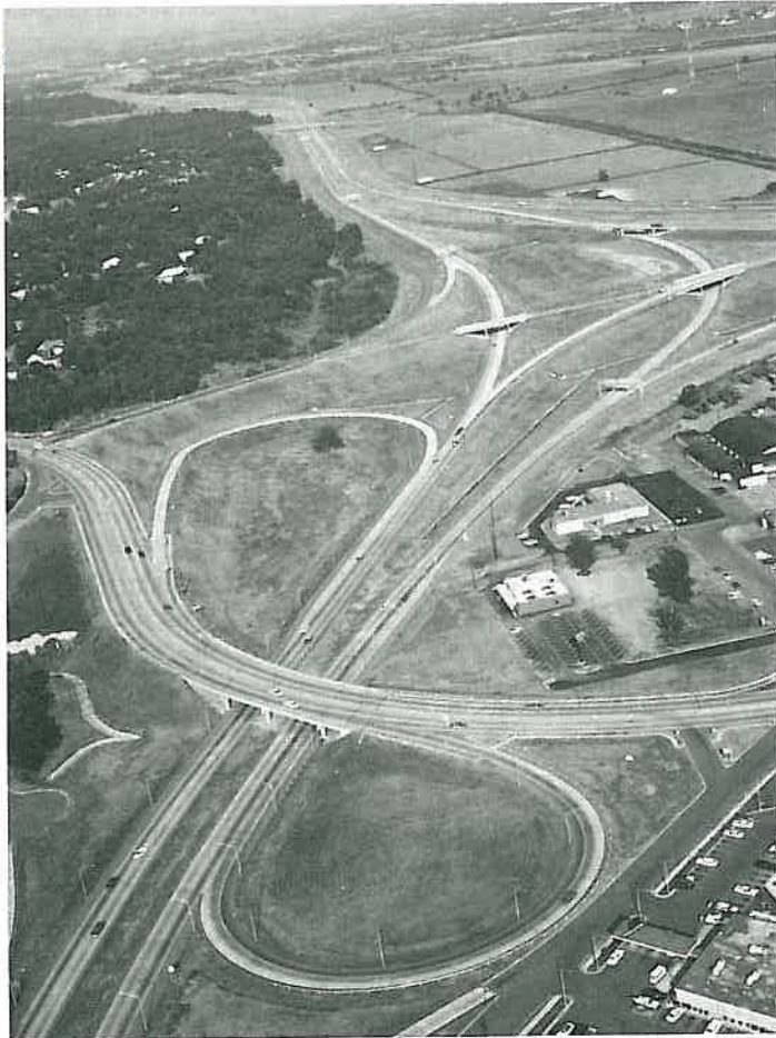
I-40/Highway 107 Overpass Looking East, 1963.
