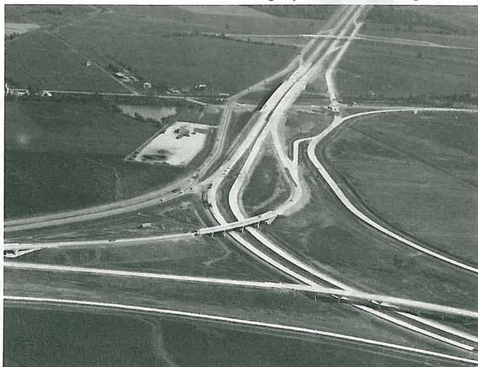
The I-55/I-40 Interchange at West Memphis in 1960.
